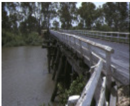
chinamans bridge over goulburn river nagambie siding detail dec1987
