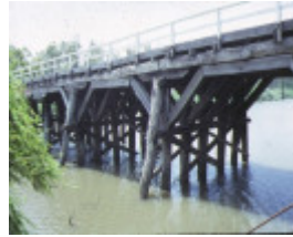
1 chinamans bridge over goulburn river nagambie side elevation dec1987
