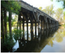
CHINAMANS BRIDGE SOHE 2008
