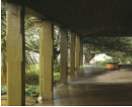
1 elderslie barringo new gisborne view of verandah
