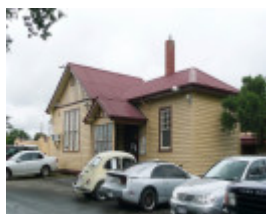
NEW GISBORNE RAILWAY STATION COMPLEX SOHE 2008
