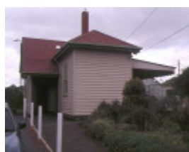
new gisborne railway station complex station road side elevation apr1995
