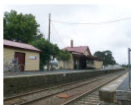
NEW GISBORNE RAILWAY STATION COMPLEX SOHE 2008
