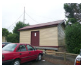
NEW GISBORNE RAILWAY STATION COMPLEX SOHE 2008
