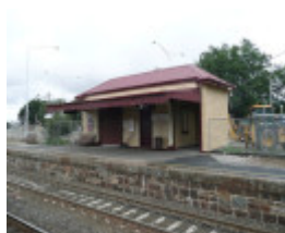
NEW GISBORNE RAILWAY STATION COMPLEX SOHE 2008
