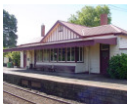
Gisborne Station Building
