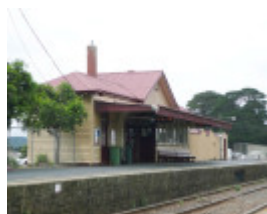
NEW GISBORNE RAILWAY STATION COMPLEX SOHE 2008
