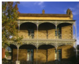
armytage house pakington street newtown side view 1997
