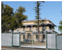
ARMYTAGE HOUSE SOHE 2008
