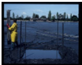
ALBERT PARK LAKE EXCAVATION
