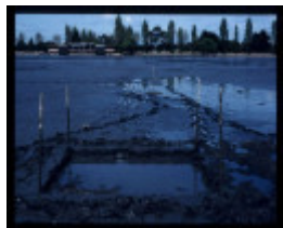
ALBERT PARK LAKE EXCAVATION
