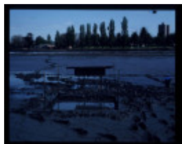
ALBERT PARK LAKE EXCAVATION
