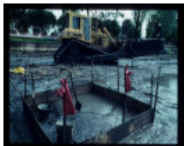
ALBERT PARK LAKE EXCAVATION
