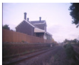
bannockburn railway station side view apr1995
