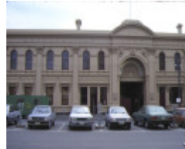
former metropolitan meat market nth melb external entrance
