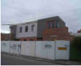
carlton north ogrady street carlton north ogrady street 12
