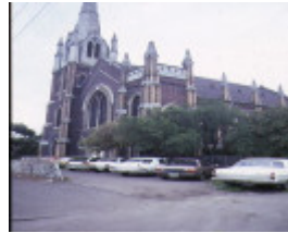
presbyterian church north melb exterior front
