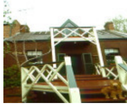
596 queensbury street rear august 2000
