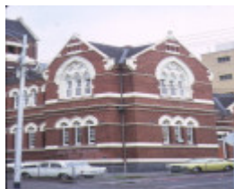
melbourne college of printing & graphic arts queensberry street north melbourne corner view mar1985
