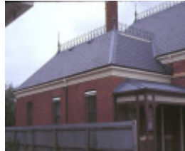
numurkah court house melville street numurkah side elevation nov1984
