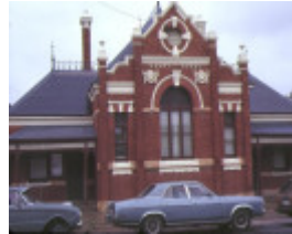
1 numurkah court house melville street numurkah front view nov1984
