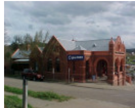
former omeo post office corner view oct1999
