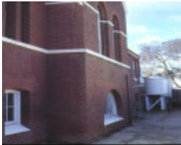
former omeo post office side wall jul1980
