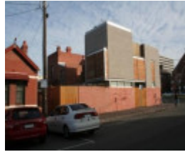
Rear of 286 Rathdowne Street.JPG
