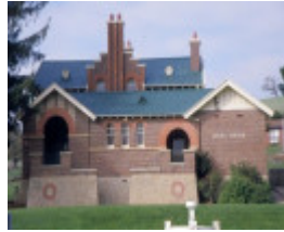
h01536 1 omeo justice precinct day avenue omeo 1893 courthouse from day avenue
