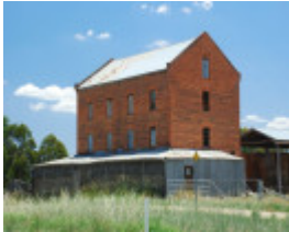
FORMER FLOUR MILL SOHE 2008
