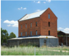
FORMER FLOUR MILL SOHE 2008
