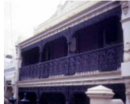
h00086 1 mentone park drive parkville verandah
