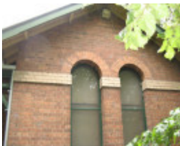
segmental arched window pair to facade
