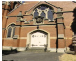
presbyterian college church royal prd parkville detail front entrance jan1997
