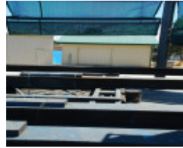
SLIP AND WINCH SHED SOHE 2008
