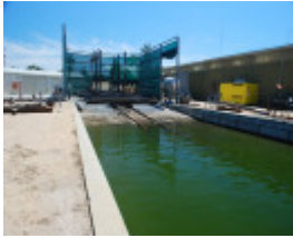
SLIP AND WINCH SHED SOHE 2008
