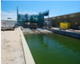
SLIP AND WINCH SHED SOHE 2008
