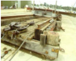
h01648 1 government slipway paynesville slip detail nov1998
