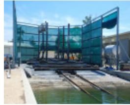
SLIP AND WINCH SHED SOHE 2008
