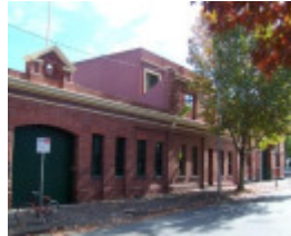
Cable Tram Engine House
