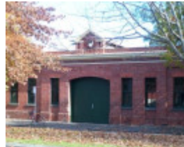
Cable Tram Engine House
