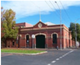
Cable Tram Engine House
