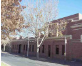
Cable Tram Engine House - 1023 Rathdowne
