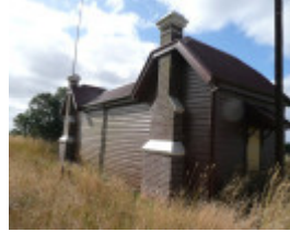
PIRRON YALLOCK RAILWAY STATION COMPLEX SOHE 2008
