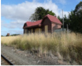
PIRRON YALLOCK RAILWAY STATION COMPLEX SOHE 2008
