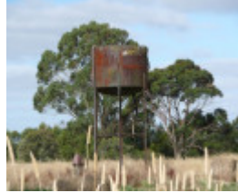
PIRRON YALLOCK RAILWAY STATION COMPLEX SOHE 2008
