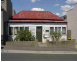
richmond waverley street richmond waverley street 11
