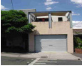
richmond waverley street richmond waverley street 13a
