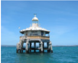
SOUTH CHANNEL PILE LIGHT SOHE 2008
