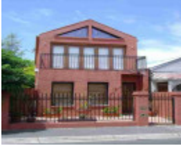
richmond woodlawn street richmond woodlawn street 15
