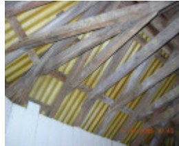
WEST CHANNEL PILE LIGHT SOHE 2008
