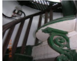
WEST CHANNEL PILE LIGHT SOHE 2008
