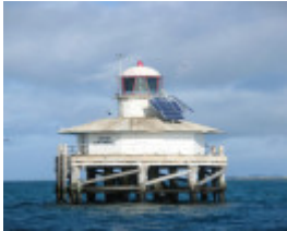
WEST CHANNEL PILE LIGHT SOHE 2008
