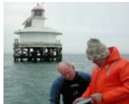
h01518 west channel pile light brad and lyall
