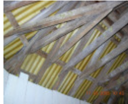
WEST CHANNEL PILE LIGHT SOHE 2008
