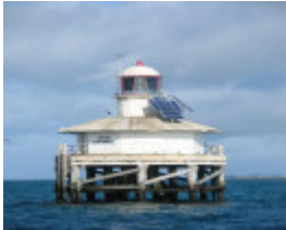
WEST CHANNEL PILE LIGHT SOHE 2008
