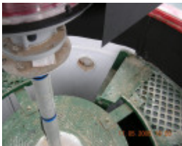
WEST CHANNEL PILE LIGHT SOHE 2008
