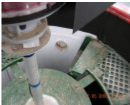
WEST CHANNEL PILE LIGHT SOHE 2008
