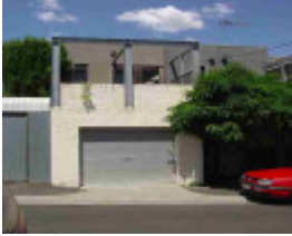
richmond waverley street richmond waverley street 25
