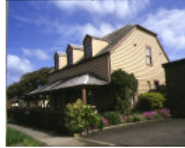
1 former steampacker hotel front view
