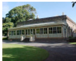
burswood cape nelson road portland front view nov1999
