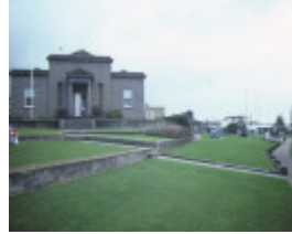
1 portland court house cliff street portland front view may1984
