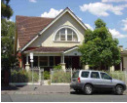
richmond docker street richmond docker street 25-27
