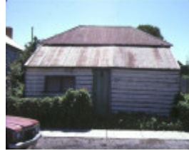
1 dwelling 8 glenelg street portland front view
