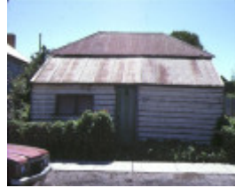
1 dwelling 8 glenelg street portland front view
