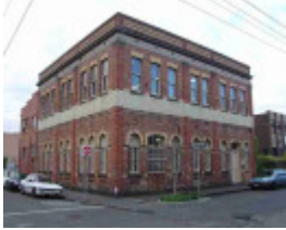
fitzroy argyle street fitzroy argyle street 71
