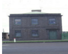
1 residence 70 julia street portland front view
