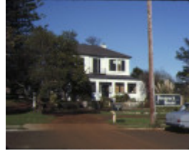
1 prospect portland front view from street
