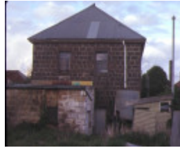
1 jay's laundry portland rear view
