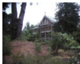
belmont raglan rd beaufort rear view house mar1985
