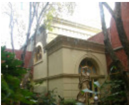
Prahran Town Hall NE Corner Council Chambers 2 May 05
