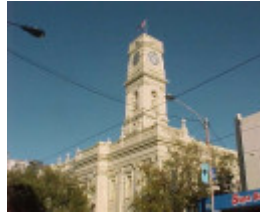
h00203 prahran town hall greville street prahran clock tower she project 2004
