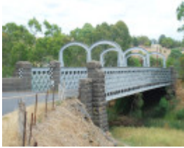
Redesdale Bridge aerial view
