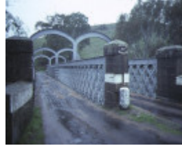
1 Redesdale Bridge redesdale end of bridge
