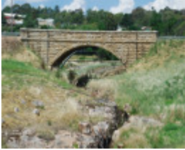
NEWTOWN BRIDGE PRECINCT SOHE 2008
