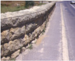
newtown bridge precinct beechworth side wall of bridge
