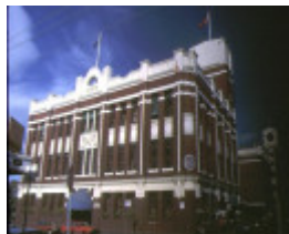
1 former bryant & may industrial complex church street richmond front view nov1984
