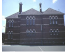
1 primary school number 2084 cremorne street richmond rear elevation nov1984
