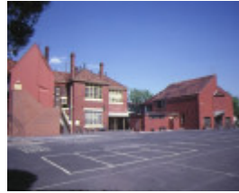
Primary School No. 2798, Davison Street Richmond, rear view, Nov 1984
