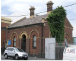
FORMER GAS INSPECTOR'S RESIDENCE SOHE 2008
