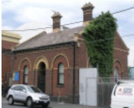
FORMER GAS INSPECTOR'S RESIDENCE SOHE 2008
