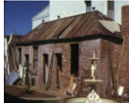
1 former cbc bank camp street beechworth servant's quarters
