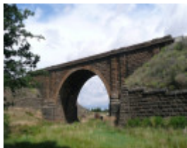
RAIL BRIDGE SOHE 2008
