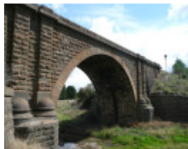
RAIL BRIDGE SOHE 2008
