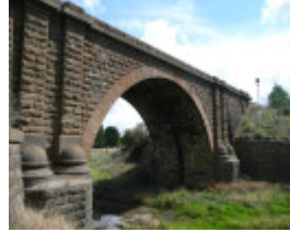
RAIL BRIDGE SOHE 2008
