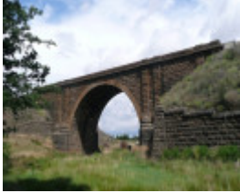
RAIL BRIDGE SOHE 2008
