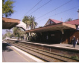
1 ripponlea railway station complex glen eira road riponlea upside building aug1998
