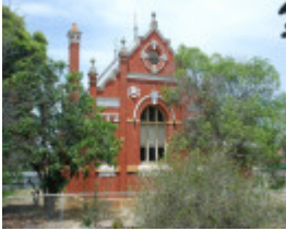
ROCHESTER COURT HOUSE SOHE 2008
