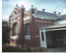
1 rochester court house rochester front elevation jul1984
