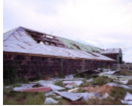
1 deanside woolshed complex rockbank exterior of woolshed
